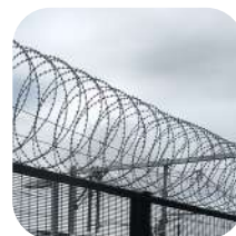
Razor Wire (Installed on top)
